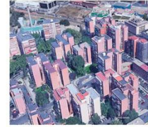
HT : Housing tower
